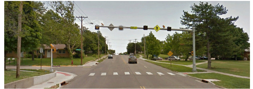
Pedestrian intersection improvements at Fisher Street and 47th Avenue, such as this enhancement of the warning signs with pedestrian actuated flashing beacons mounted overhead is recommended to improve pedestrian safety.
