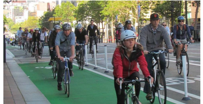
Protected bicycle lanes, such as the one in the photo, provide physical separation between cars and cyclists. Protected bicycle lanes are safer, and have been shown to increase cycling levels by attracting people that are uncomfortable biking on the street or in conventional on-street bike lanes.
